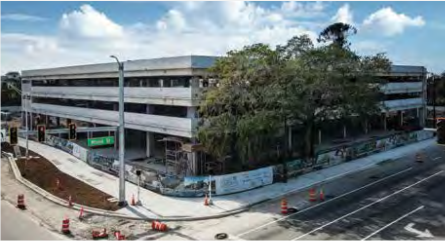
The new MURT, now open while construction continues, is made possible by the generous support of Selby Gardens Board Chair Marianne McComb and her husband, Bill.
